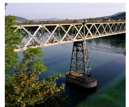
A Section of the Girder Bridge over the Rhine at Hemishofen (Switzerland) by Christian Kleis
